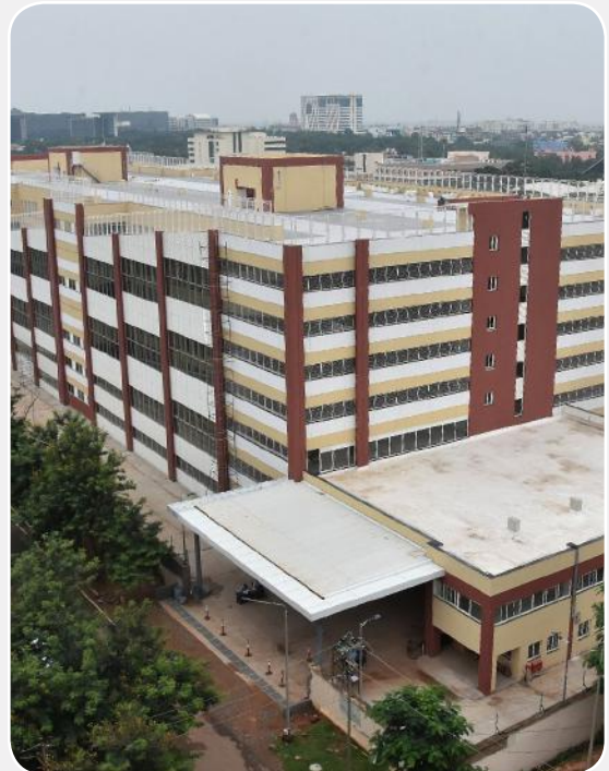
Multli Level Parking, 7-storey, Bhubaneswar, India
